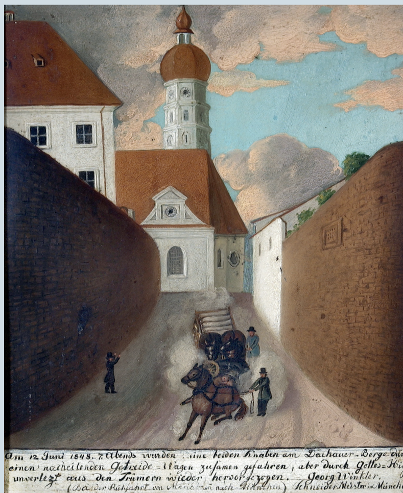
Even after modification, the road down the hill remained dangerous: On 12 June 1848, my two boys were hit on Dachau hill by a corn wain rapidly following behind, but with God’s help they were pulled from the wreckage uninjured... , votive tablet at the pilgrimage chapel of Maria-brunn (near Röhrmoos)
